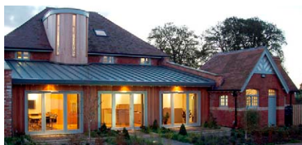
Conversion of a Coach House to commercial offices
