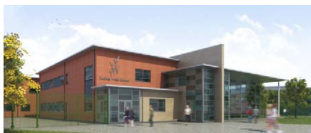
Rushey Mead school required extensive remodelling
